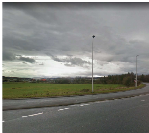
4. View North from A91 roundabout
